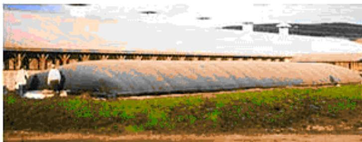
**Figure 7b.** Photo of a methane digester. It processes manure at a dairy with 800 cows, producing 775 kW of electricity. This is enough to power 600 homes.<sup>168</sup>
